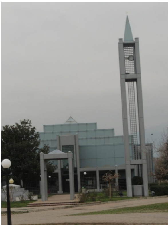
Fig. 115 Buttim Mosque, view of the minaret and kiosk.
