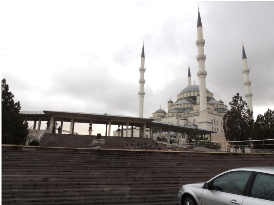
Fig. 60 General view of Kocatepe Mosque. (Photograph by Samaa Moustafa)
