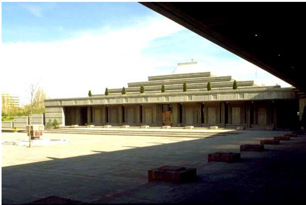
Fig. 95 Parliament Mosque, bases of columns in front of porticos.
