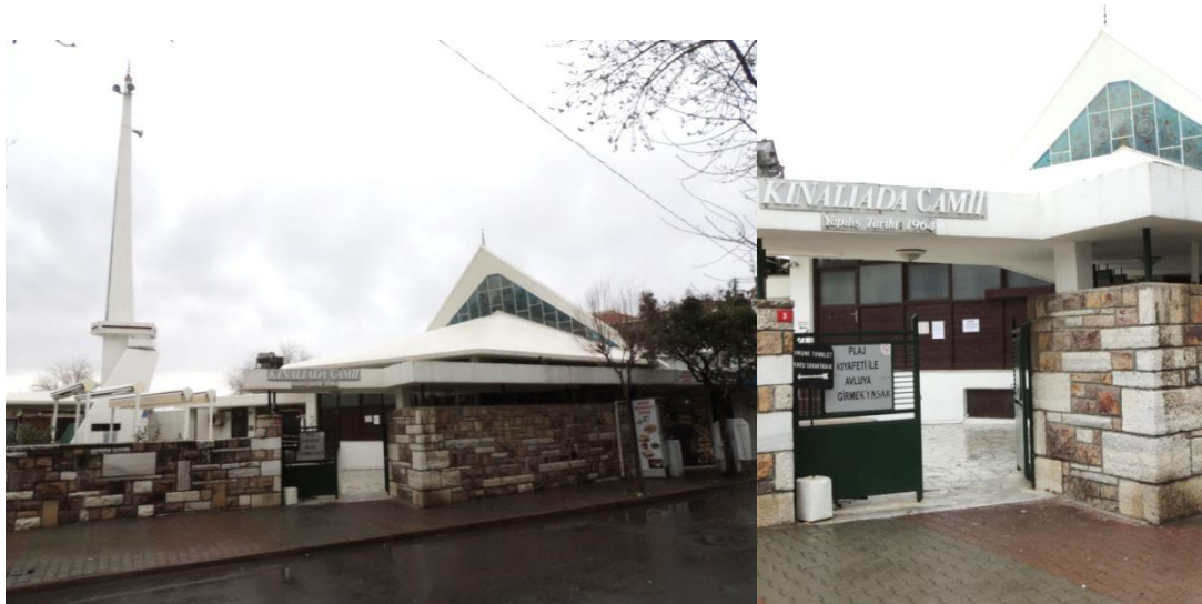
Fig. 35 Kinali Island Mosque, general view and main Entrance
