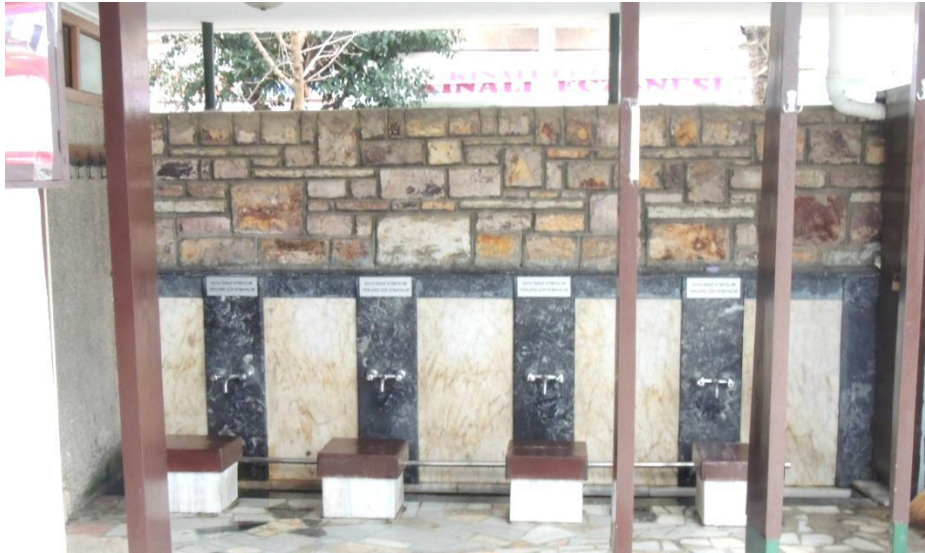
Fig. 37 Kinali Island Mosque, water taps in courtyard for ablution
