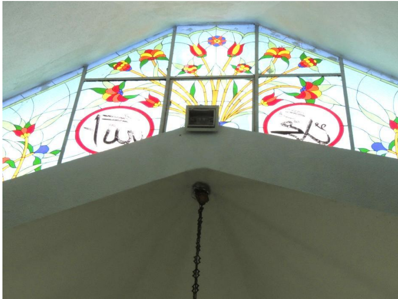
Fig. 43 Kinali Island Mosque, roof details from interior
