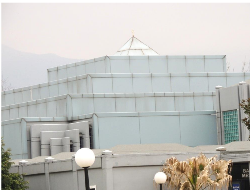
Fig. 119 Buttim Mosque, roof details of main prayer hall.
