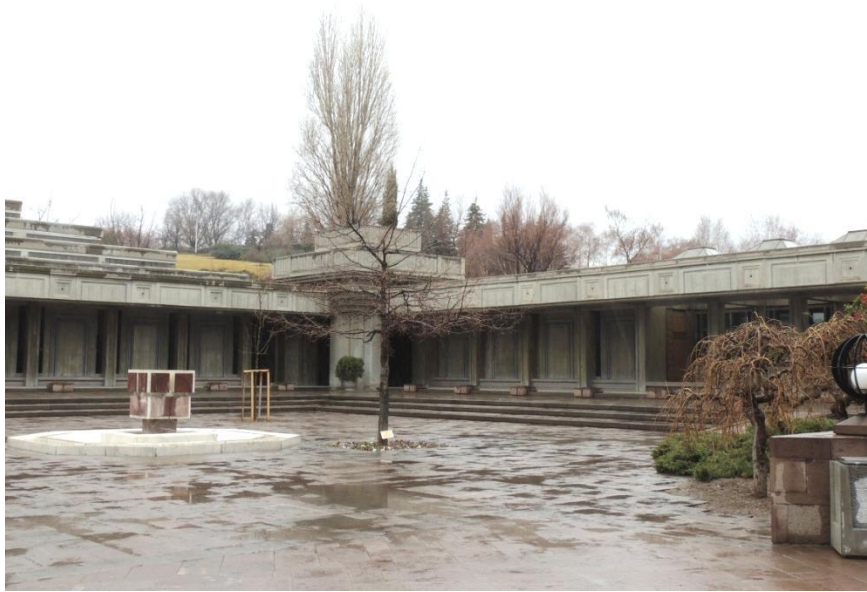
Fig. 106 Parliament Mosque, view of the minaret from forecourt.
