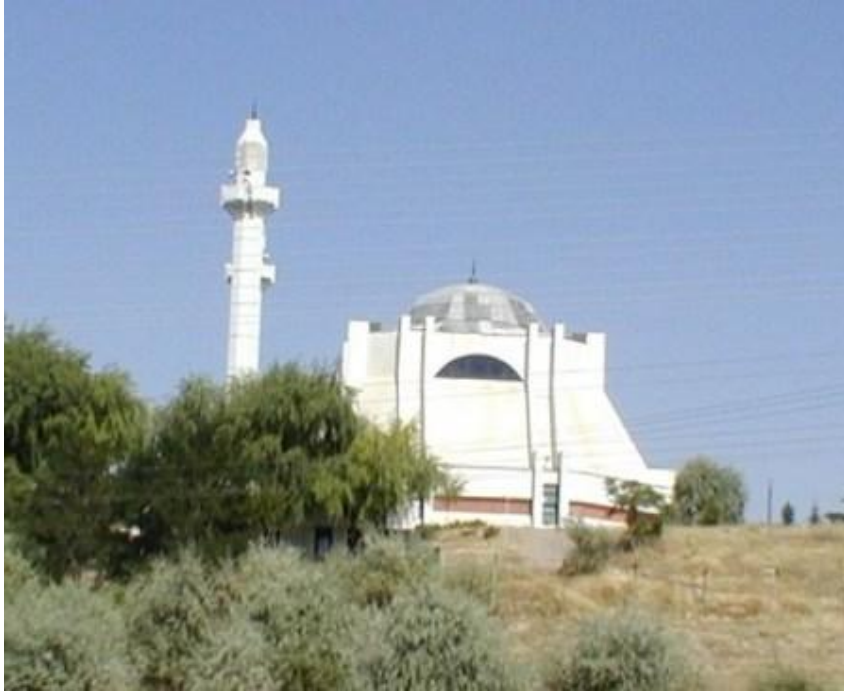
Fig. 78 TEK Mosque south façade. http://www.pbase.com .
